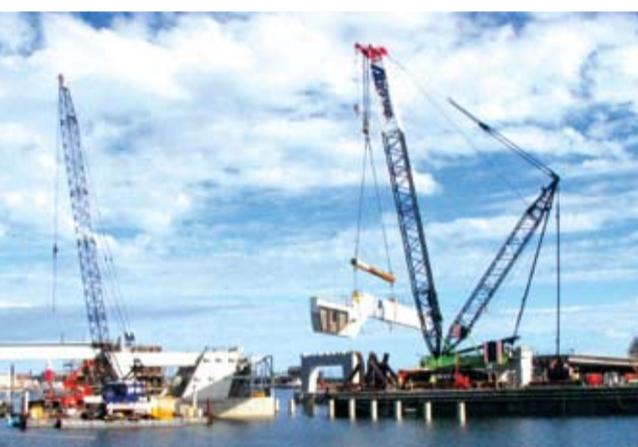
In an Australian first for a project of this scale, a shrink-fit process was undertaken to connect the rail bridge's trunnion and hub (the point at which the opening section of the bridges pivot) to the bridge girders.
