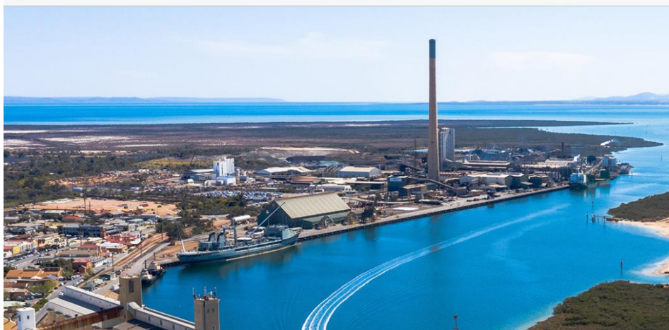
Figure 9: Pt Pirie Smelter site (Nyrstar APER, May 2022)
