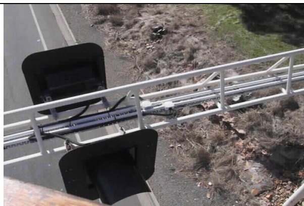
Steel truss in good condition
