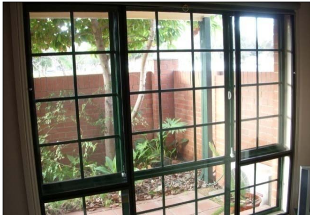
An acrylic secondary glazing system installed on the internal side of an existing window.
