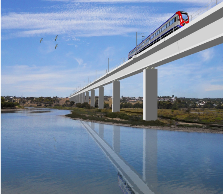
The bridge pier locations in the Onkaparinga river valley were assessed for ASS
