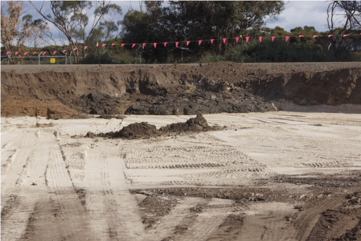
Lime placed at base of stockpile site
