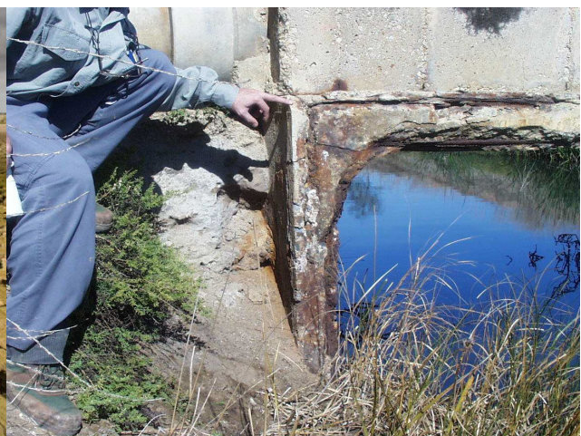
D. Impact of sulfuric material on engineered structures
