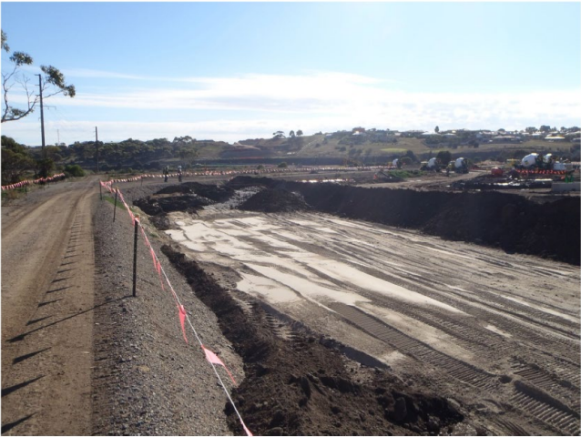
Stockpile site for ASS to be treated with lime
